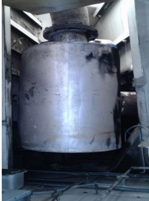
BT Silencer – side view with visual singe marks
